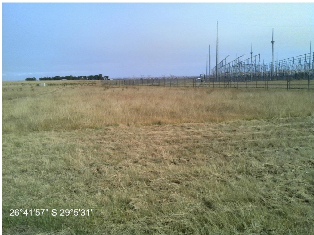
Figure 21: The Zeus Substation in the Highveld Grassveld biome.
