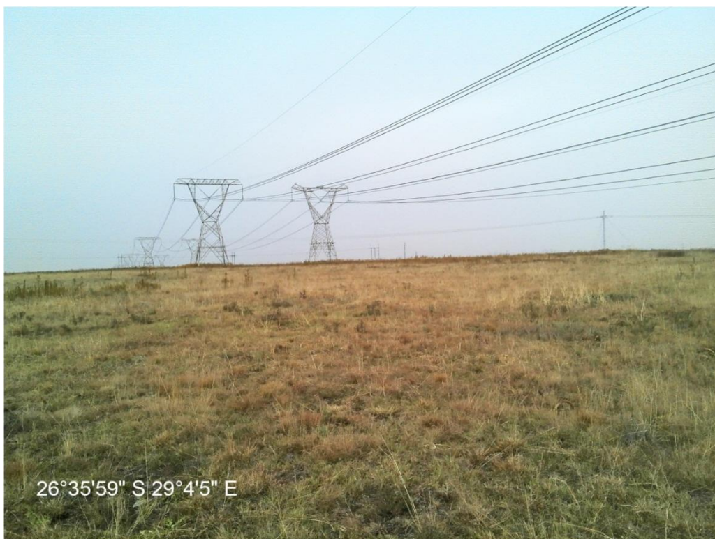
Figure 17: Grazing on turf just north of extensive maize fields. Here the new line will be to the east (right) in the servitude of the existing two lines pictured. There is less tilling in the clay soils of the southerly Soweto Highveld Grassland than on the northerly Eastern Highveld Grassland vegetation units.
